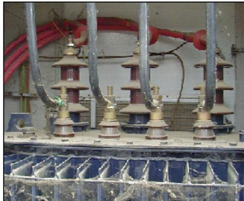
CONEXIONES TRAF0: PASATAPA S DE MT/BT CON CONEXIONES ROSCADAS DESNUDAS
